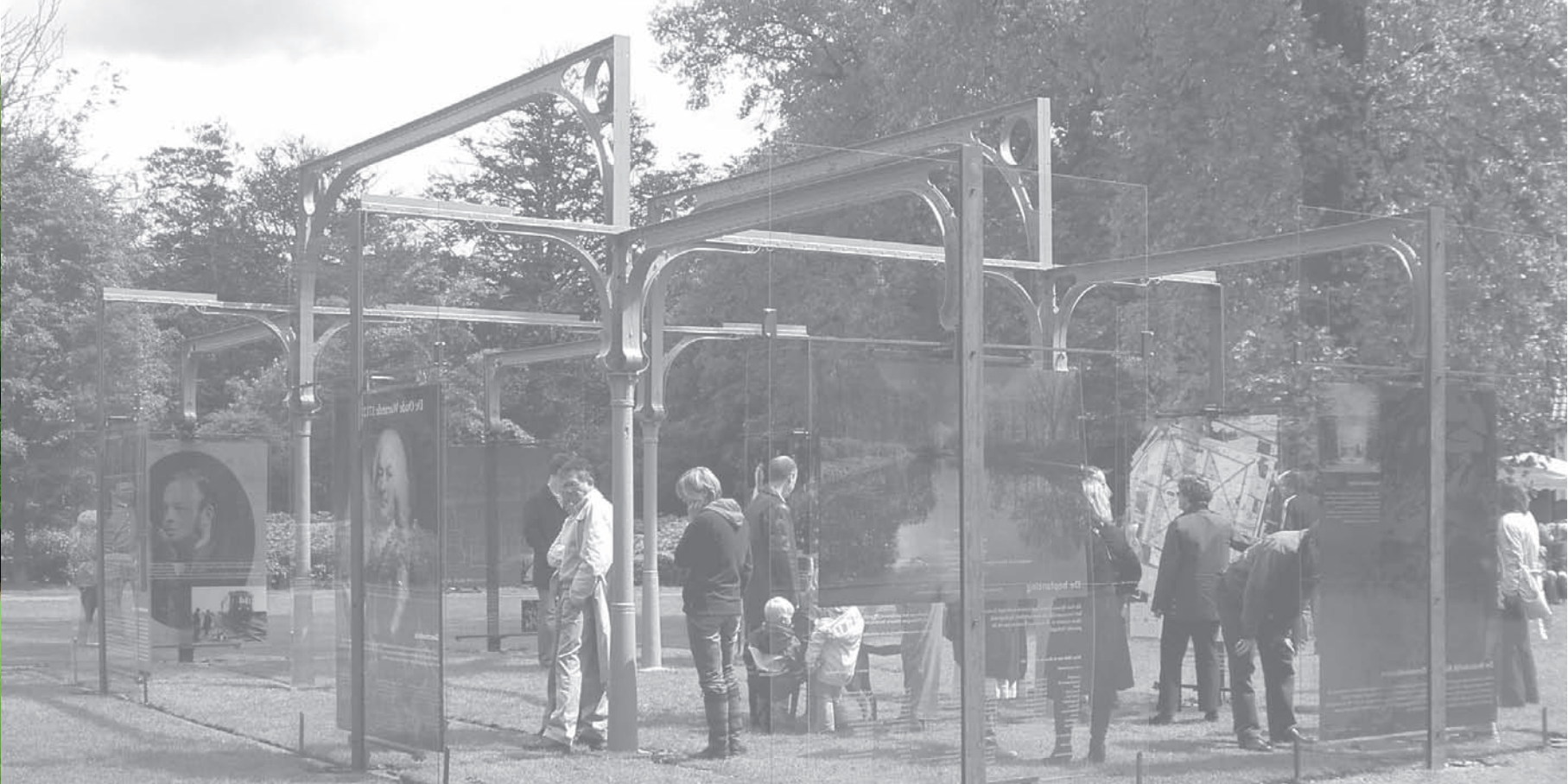
the exhibition pavilion oude warande is designed for the park holiday. jan doms made use of parts of an historical steel construction originating from the city of leuven, belgium. the exhibition of the history and restoration of oude warande is printed on hardened glass panels. tilburg local authority commissioned dr. pamela doms to carry out spatial research in the area of oude warande.
